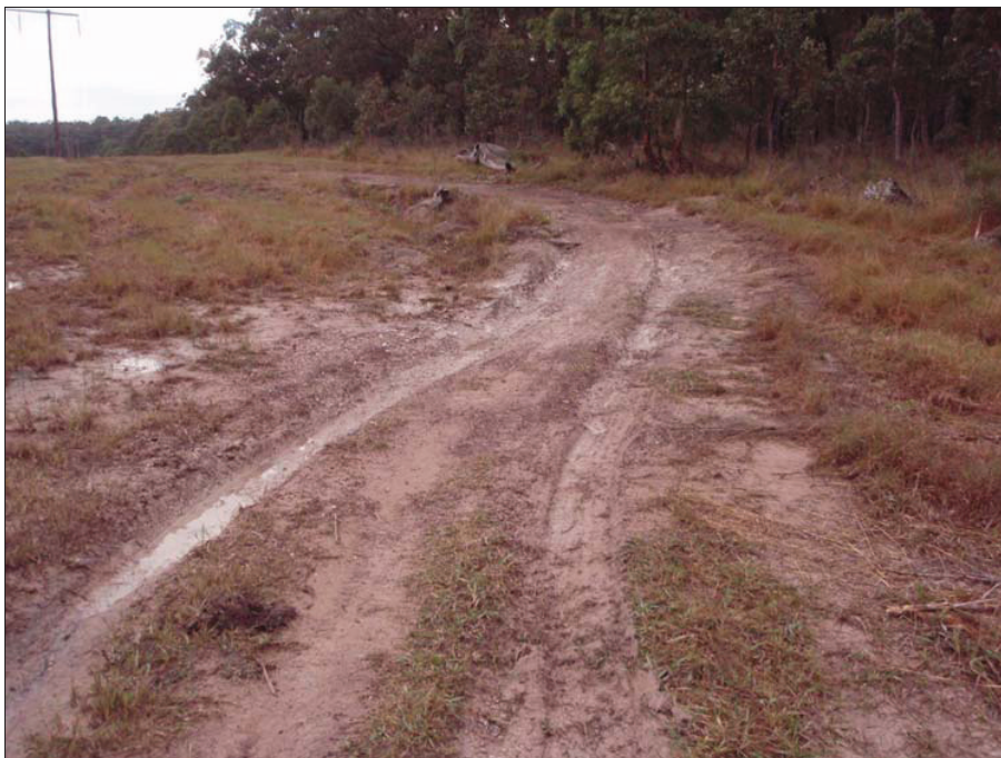
Photo 2 Exposure in track way T2 easement facing north east
